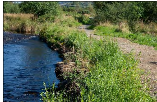
Muck Water After: The footpath is now protected, the silt/sediment input has stopped and juvenile fish have better bankside cover/refuge.
