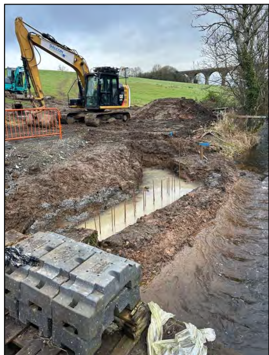
Figure 2: Purclewan Burn Engineering Works - December
