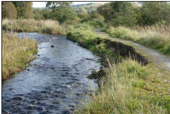
Muck Water Before: path at risk of being lost. Inputs of silt/sediment to the burn – degrading water quality.
