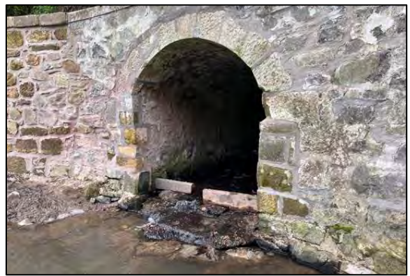
Netherton Culvert: We have now installed baffles in the culvert which should aid trout and salmon in reaching the upstream habitats that have been restored.
