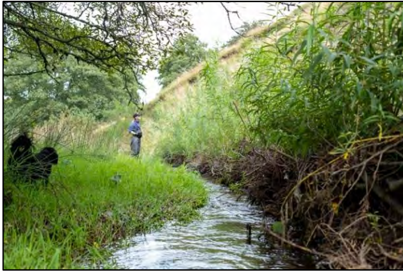
The green engineering we installed in May 2024 has transformed the toe of this sheer banking and is now helping prevent most of the alluvial soils from entering the watercourse.
