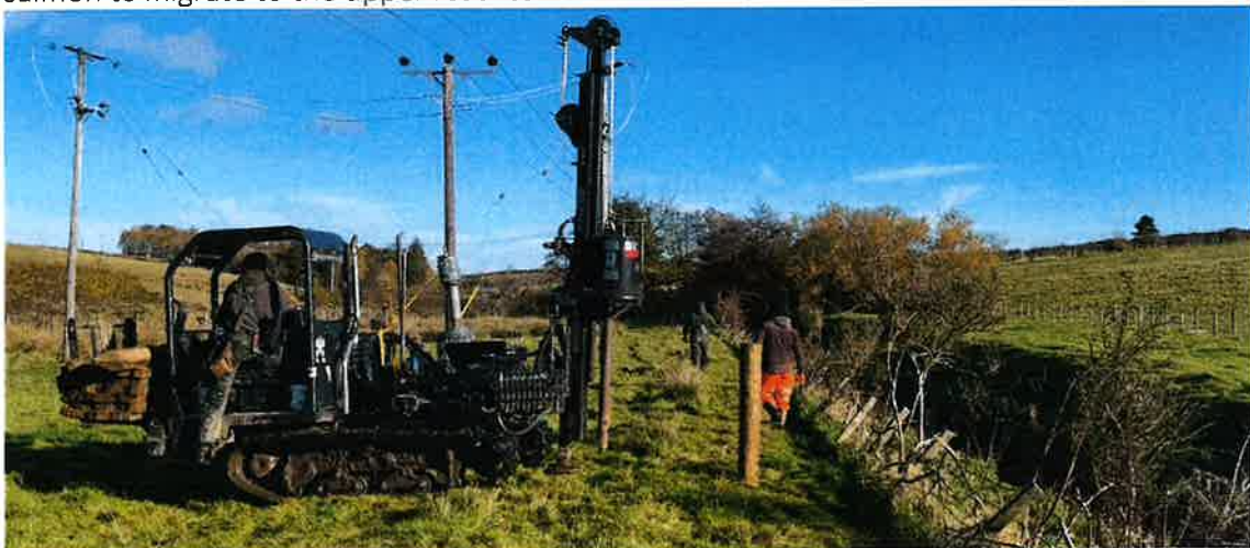
New fencing going in on Brockloch
