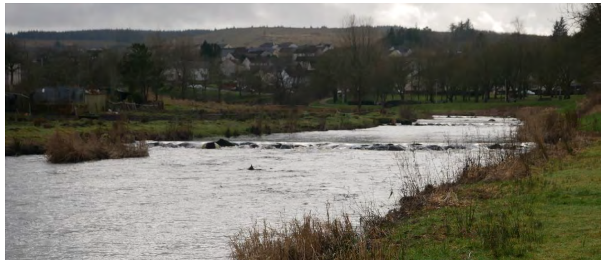
Figure 5: Water from the upper weir is backed up to these artificially stepped pools. Removing the centre sections of these dams may also be beneficial to smolts, adults and angling following easement of the weirs downstream but this will need to be determined through consultation with stakeholders.
